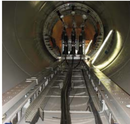
Fig. 11 - HV Cable Installation
